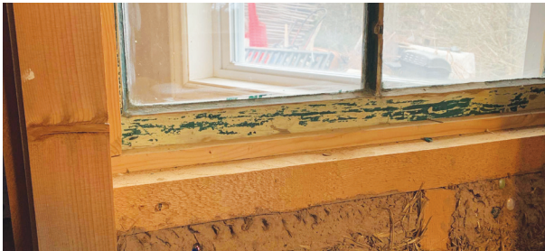
Detail of the inside of the walls at The Deanery Project -- local clay and straw
