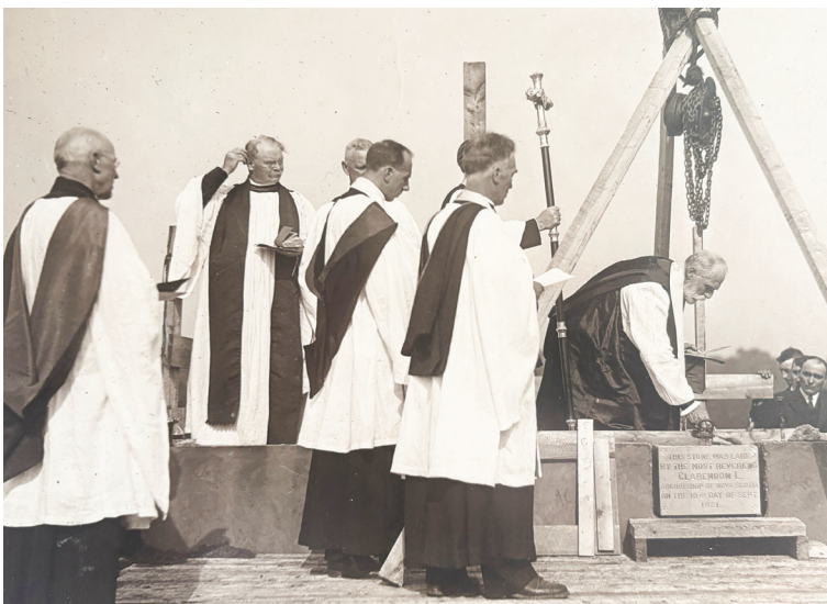
Laying the cornerstone of St. Alban's Church
