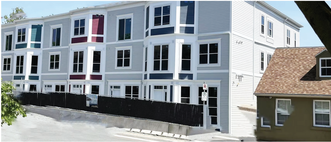
Construction of Ozanam Place, Halifax, N.S. March 2025 © ssvphalifax.ca
