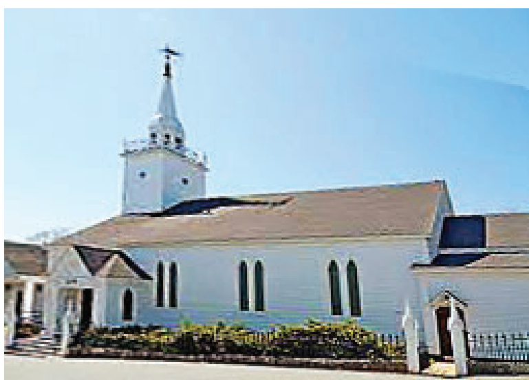
Photo: Trinity Anglican Church, Liverpool, N.S.
